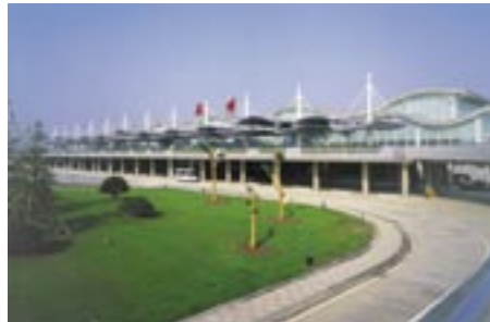
Xiaoshan International will try to utilize the experience brought by AAHK to improve operations
