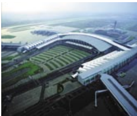
The projected three-stage "Phase Two" expansion is set to cost over RMB 7 billion
